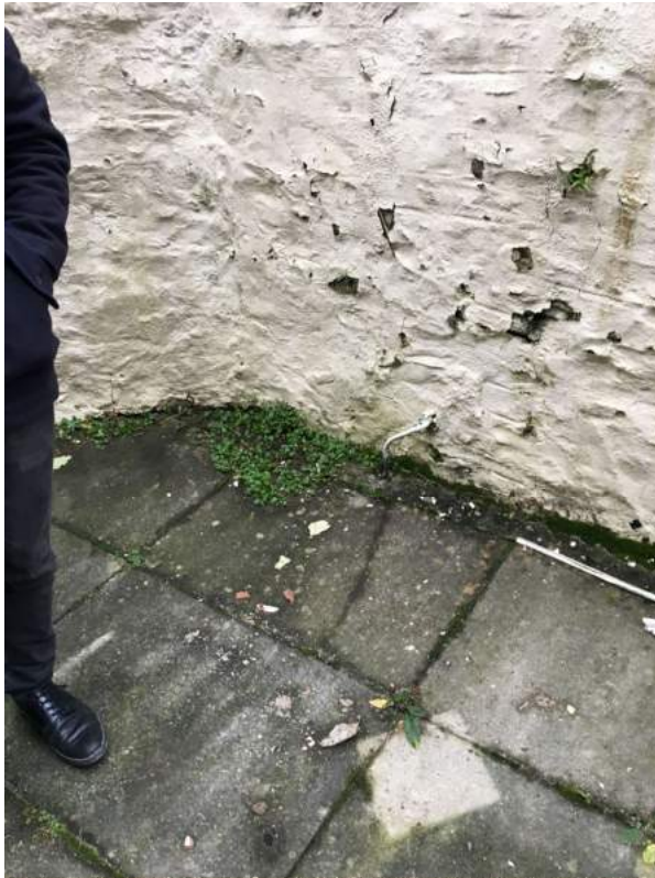
Photo 7.2.4: Existing water service heading to the cottages
