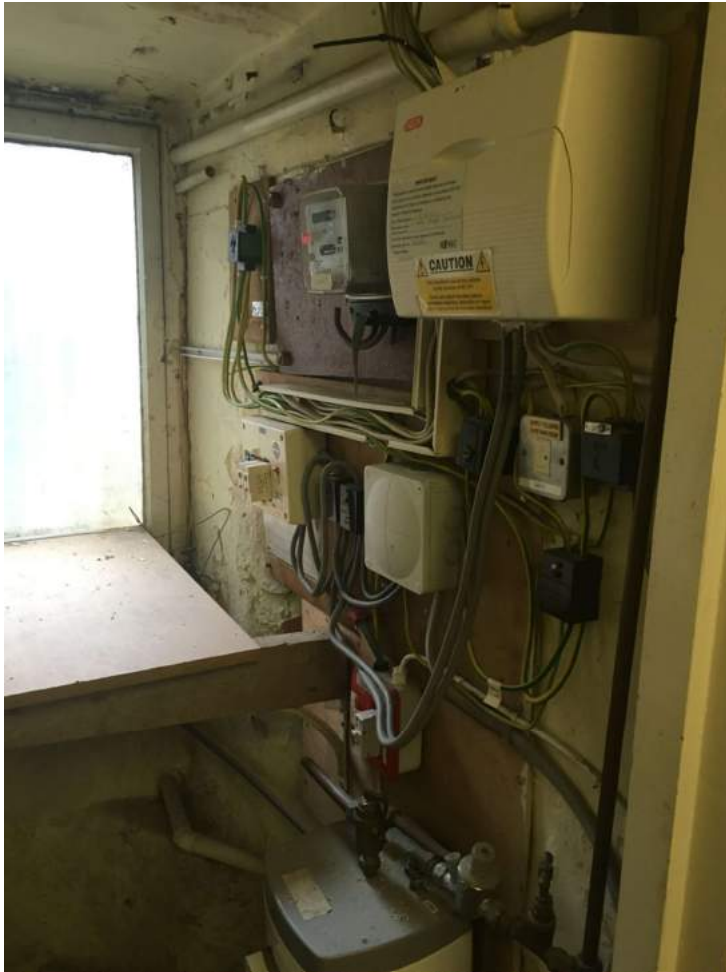
Photo 7.2.3: Existing water stop-cock cupboard (to rear of WHS Orientation space)
